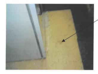
Picture 1 Floor tile stores area no asbestos was detected.
