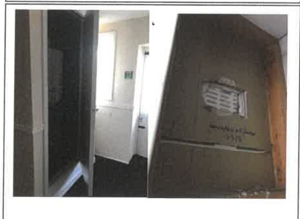
Fig 5: Boiler cupboards on first and second floor landing not suitably fire rated.
